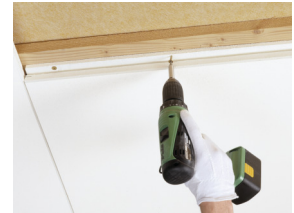
Master F is installed by screw fixing
