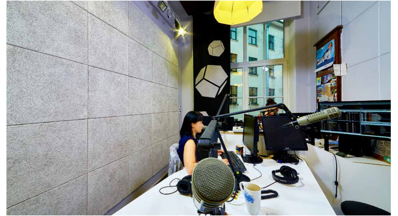
Acoustic panels provide professional soundproofing for maximum noise isolation and reduce the reflection of the sound.
