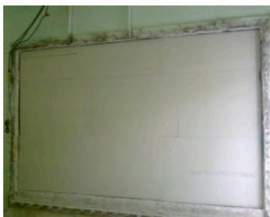
Finished wall with 12.5 mm GKB gypsum board
